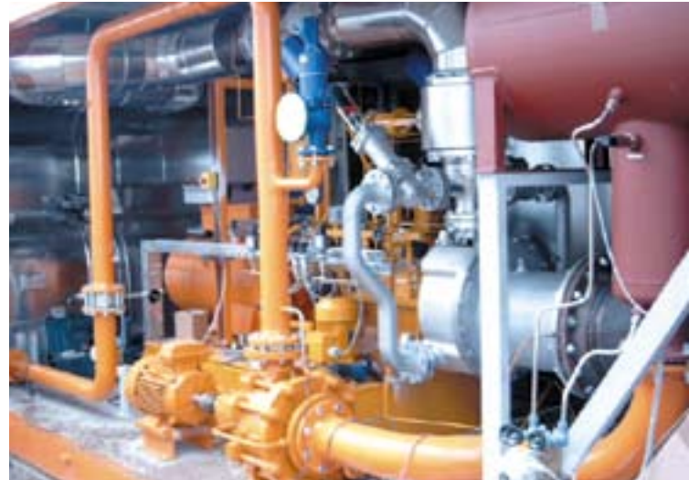
ORC (Organic Rankine Cycle) installation in the geothermal CHP plant in Newstadt-Glewe, Germany
